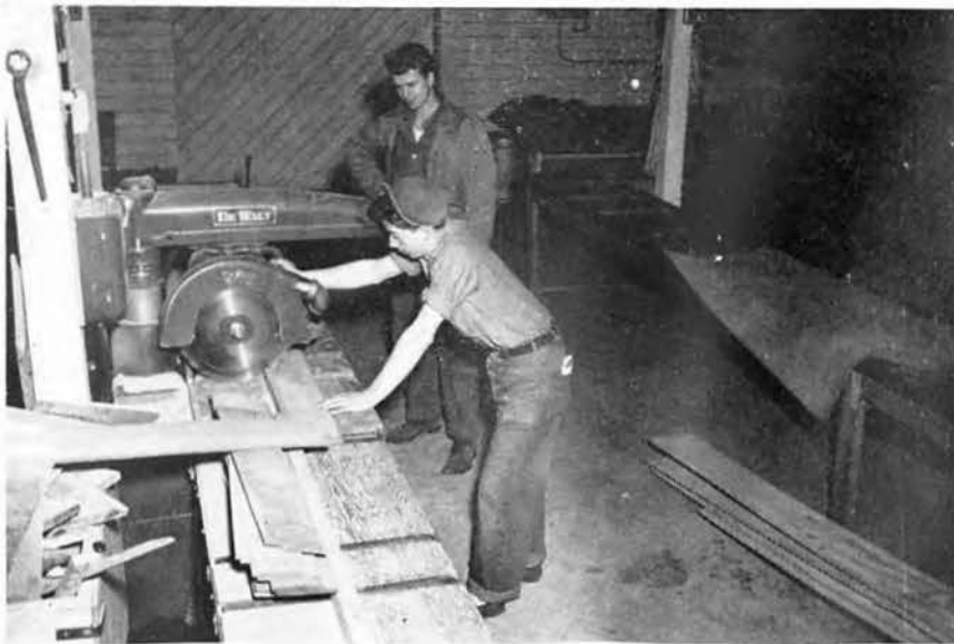
Interior of Carpenter Shop
