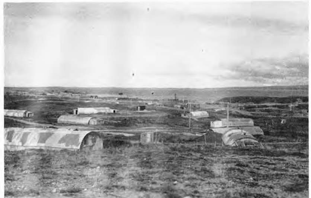
Quonset Huts Had to Be Half Buried to Withstand the Hundred Knot Winds
