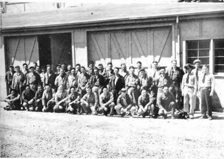
Heavy Equipment Operators and Repairmen from CB Shop
