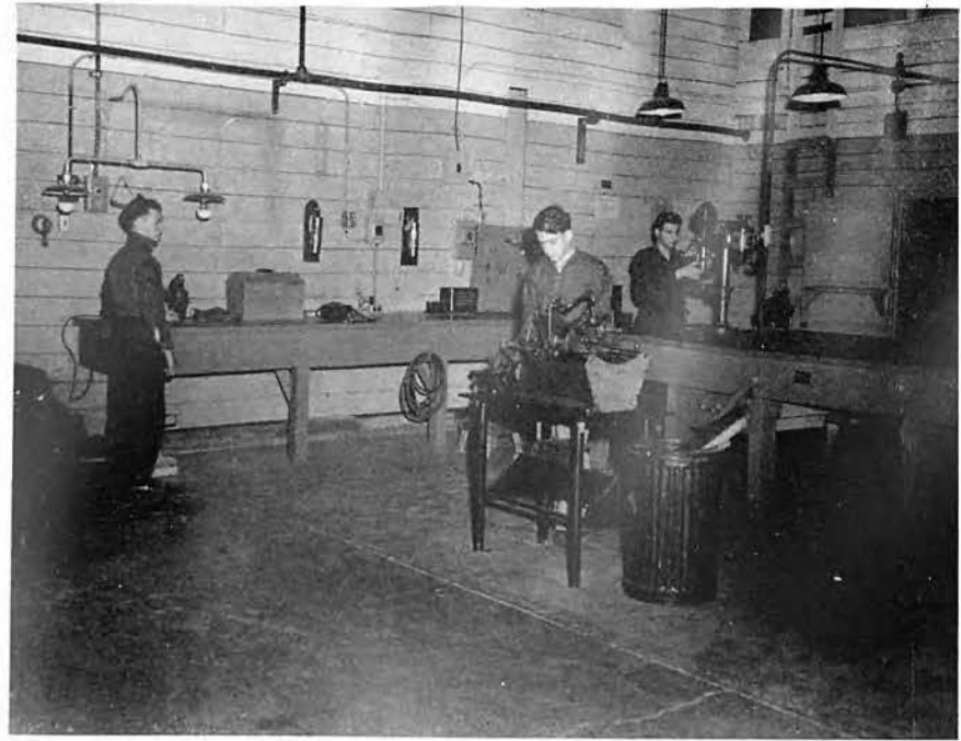
Another View of the Electric Shop
