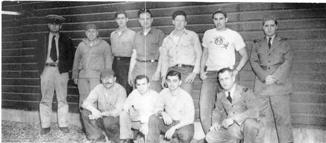
Sub Base Power Plant Crew
