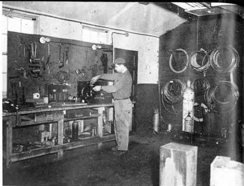
Refrigerator Repair Shop
