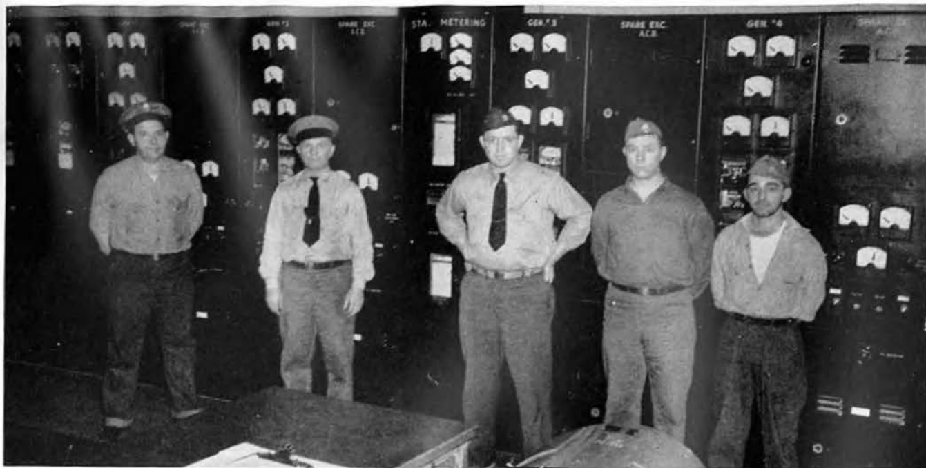
OINC and Chiefs — NOB Power Plant
