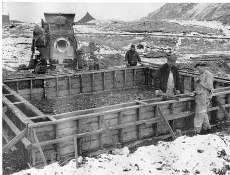
Generator Building Foundation Forms Set and Ready to Pour
