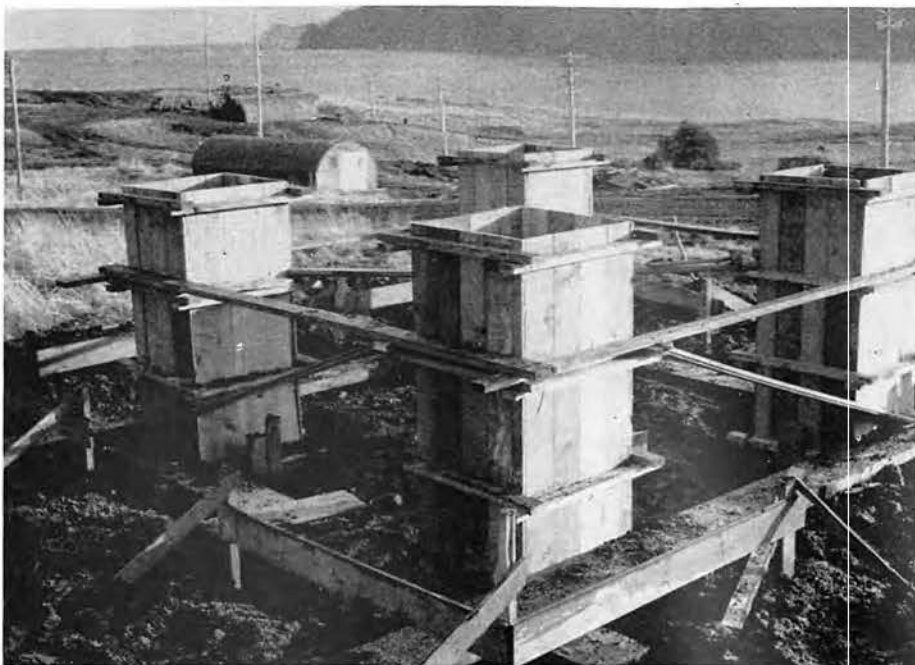
Ready to Pour Concrete Piers for North Tower
