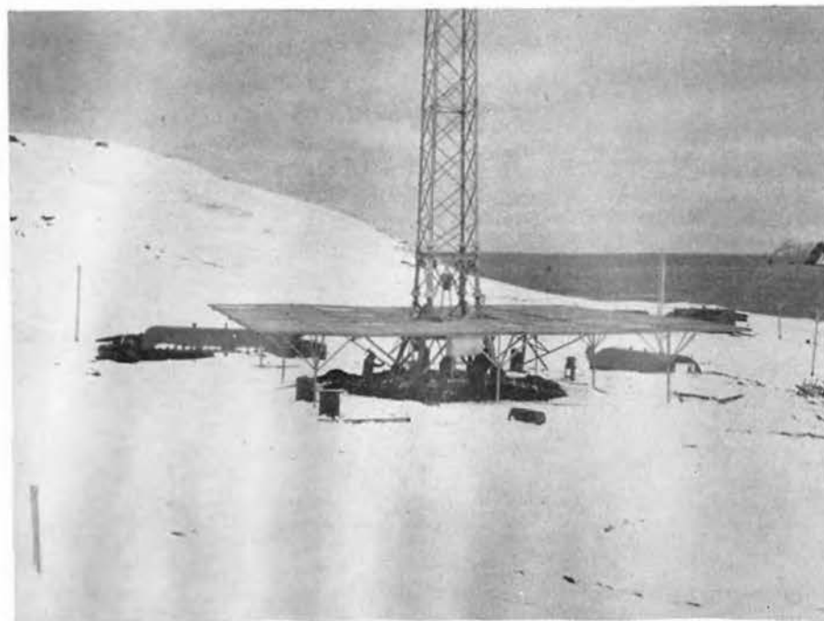
Laying the Grounding System
