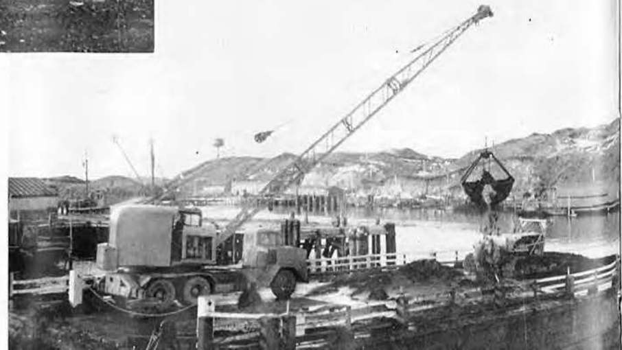
Dredging Ferry Channel Between Dutch Harbor and Unalaska Island
