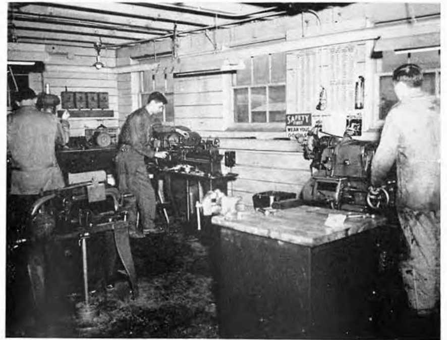
Machinists at Work in P.W. Garage Machine Shop
