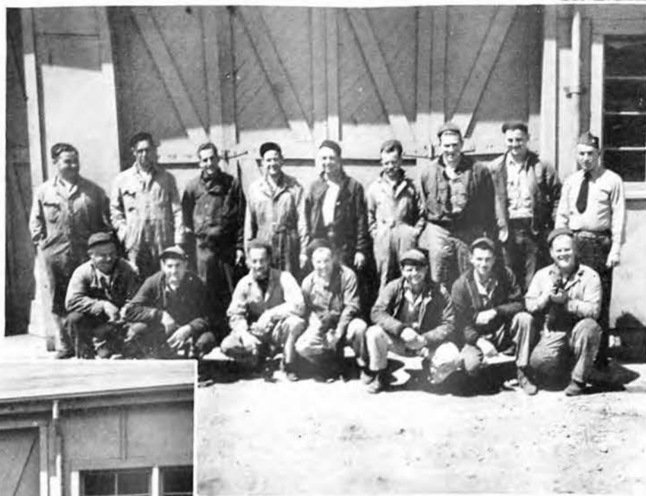
Road Maintenance of CB Shops Crew
