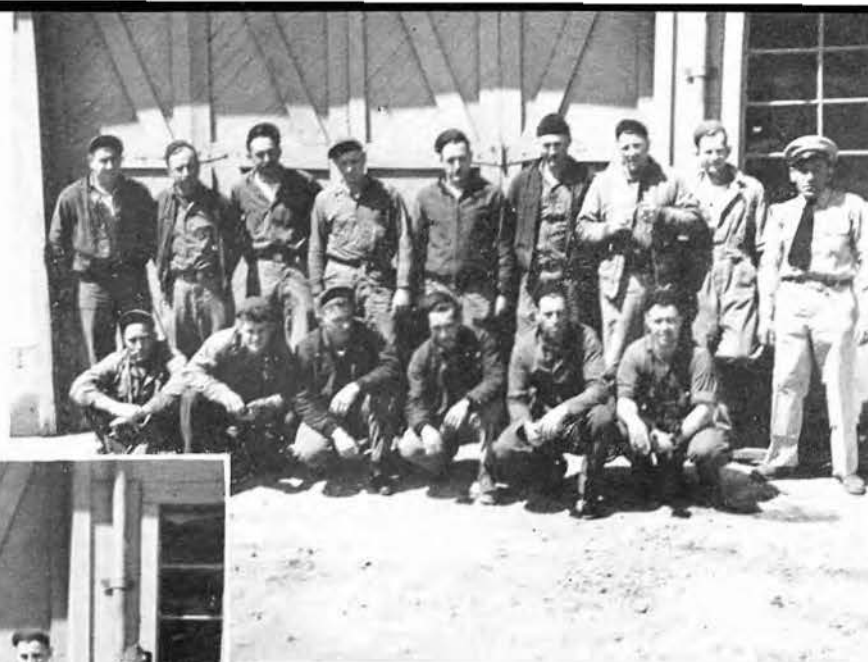
Road Maintenance Crew
