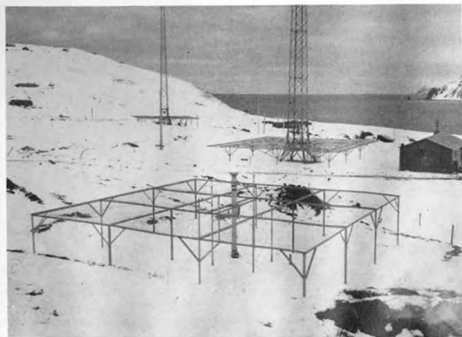
Z Marker, Radio Building, Center and North Towers Complete
