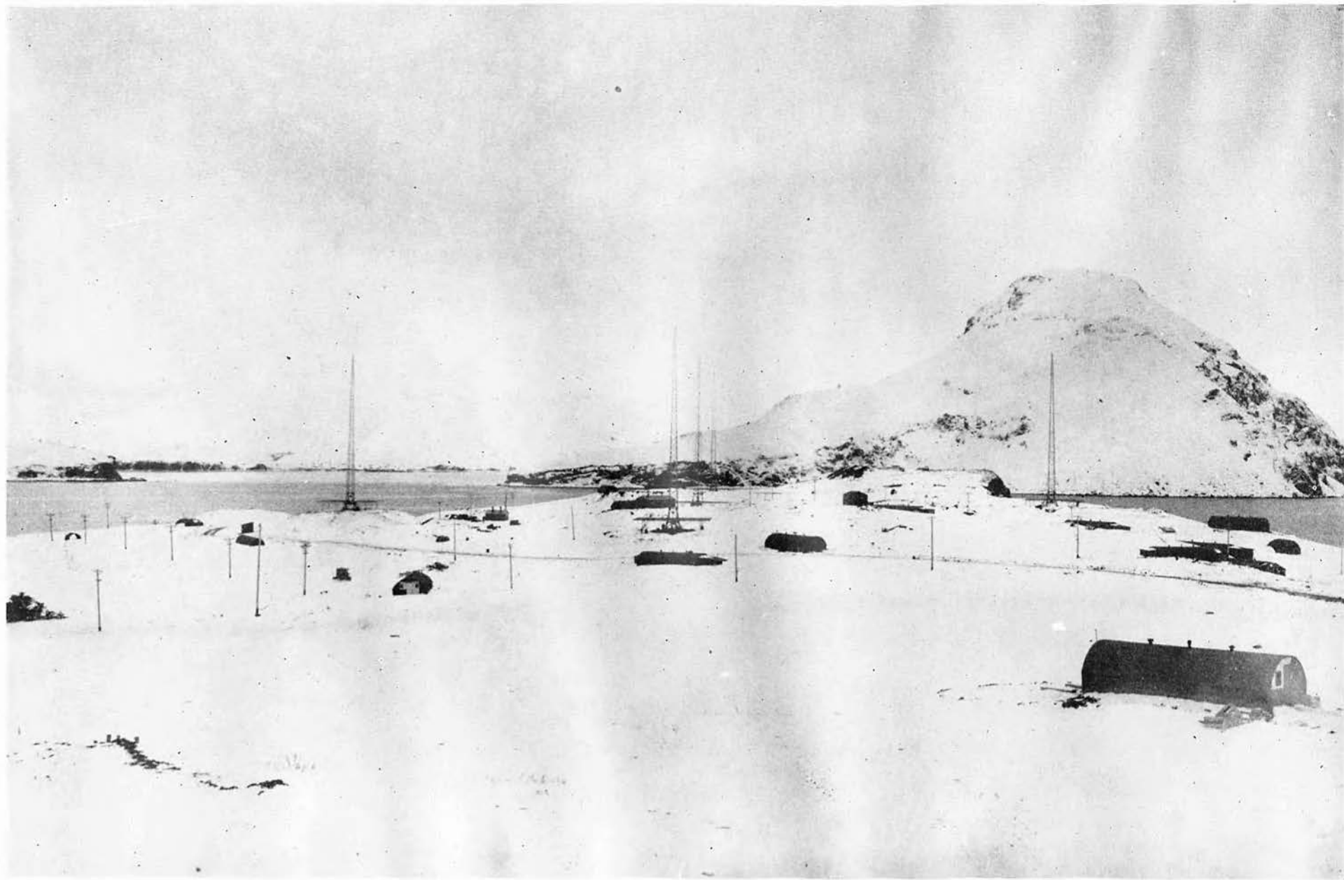
Project Completed — Overall Shot Looking Southeast, Showing Unalaska in Background
