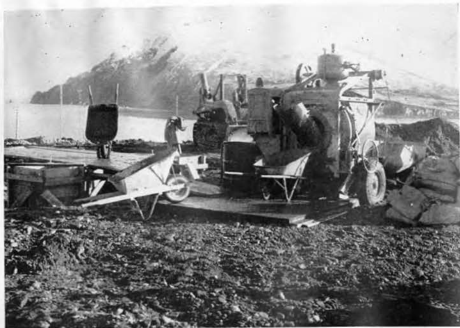
Pouring Foundation for East Tower
